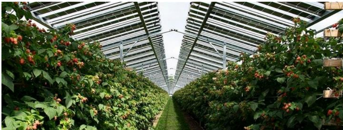
Solar installations bear fruit for Netherlands Agri-PV (case study)
